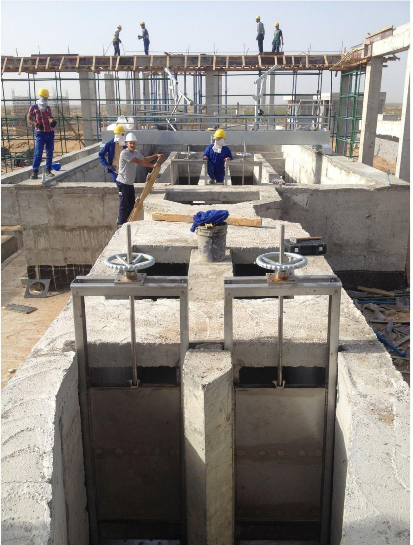
The mechanical equipments manufacturing and assembling work of “Buysanç” Gurluşyk, Babadayhan Plain 10.000 m 3 /day waste water treatment plant in Tecen Ahal Province / Turkmenistan.
